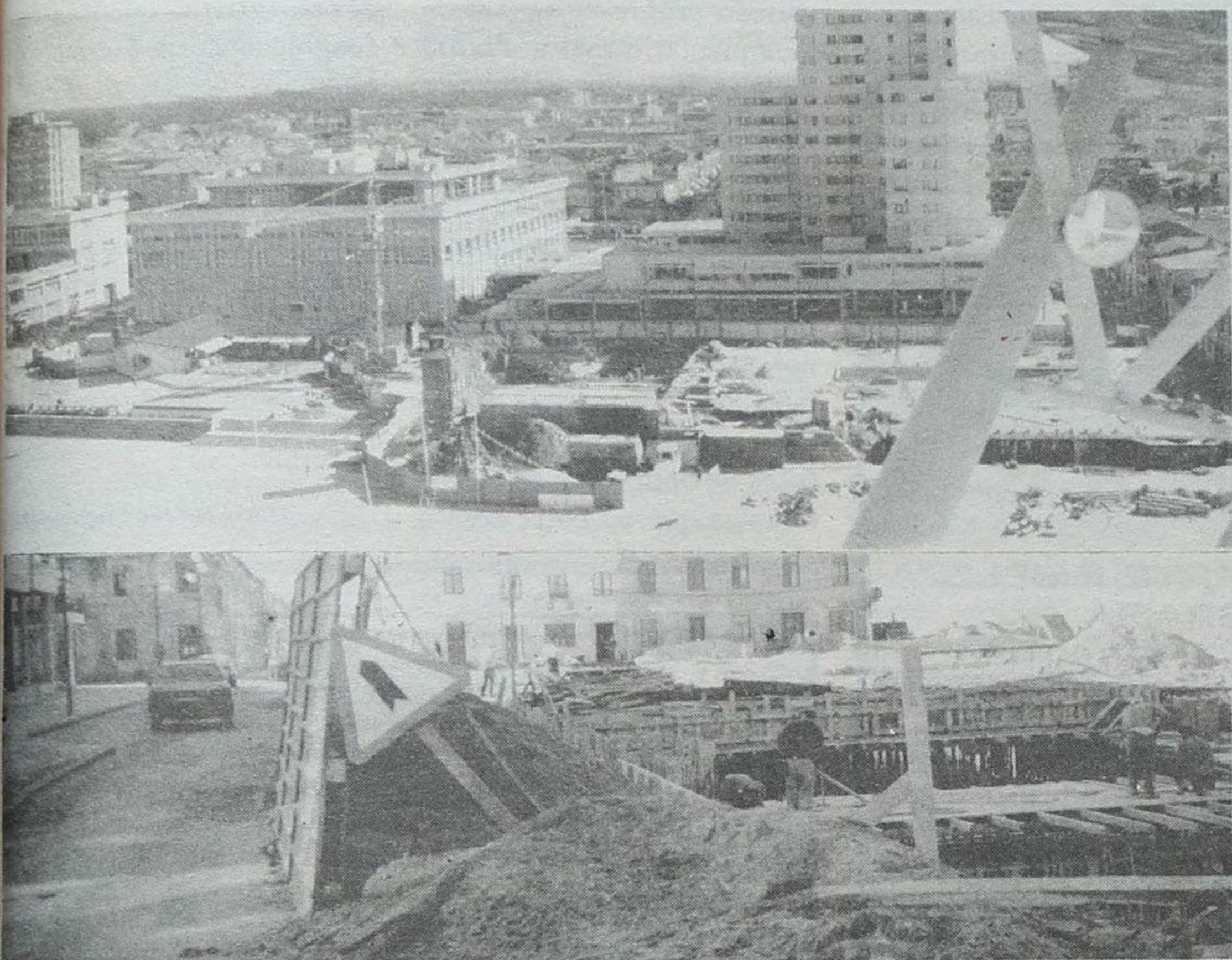
As obras no parque subterrâneo
